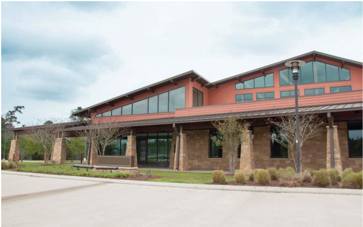
The Woodlands Township Recreation Center at Rob Fleming Park, located at 6464 Creekside Forest Drive across from The Aquatic Center at Rob Fleming Park, is open for programs, camps and events during limited hours while renovations are in progress this summer.
